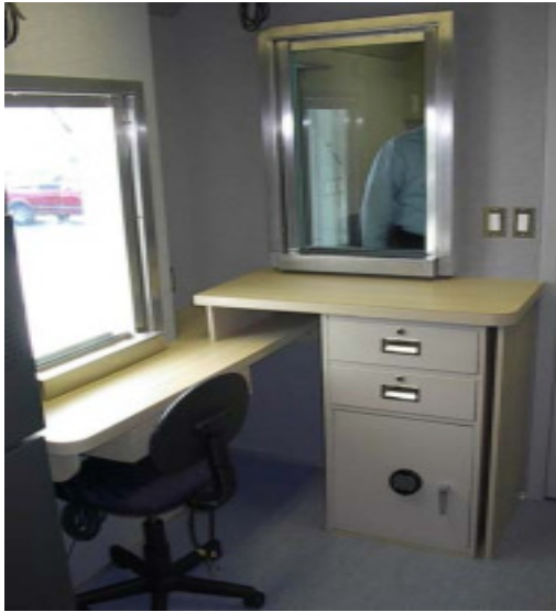
Interior & Exterior access BR glass teller windows
